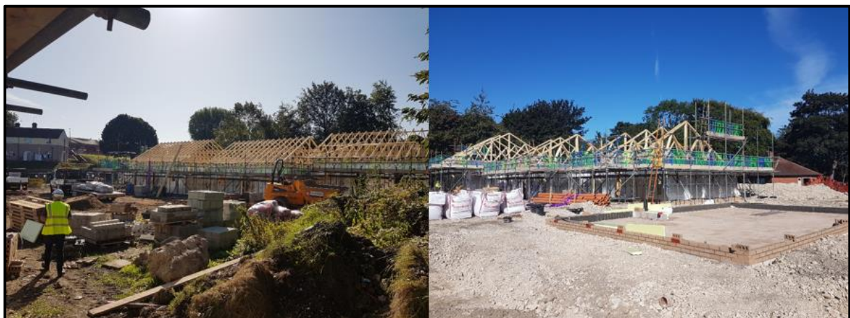
Mayman Lane: on-site progress
